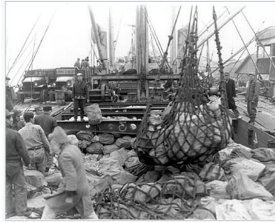
Container ships avoid the complex stevedoring of break-bulk shipping.
